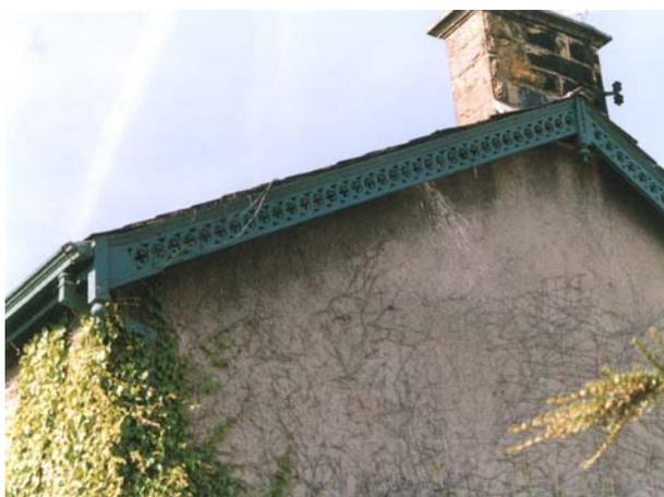
*Traditional timber gutters, and quatrefoil barge boards at the Hollies*
