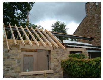
1. Trussed Rafter Roofs: these are quick to construct, measurements are taken from site and roof trusses are made up in a factory, which are delivered to site ready for installation. Each roof is individually designed by the roof truss manufacturer using specialist computer software and the carpenter's time on site can be significantly reduced.
