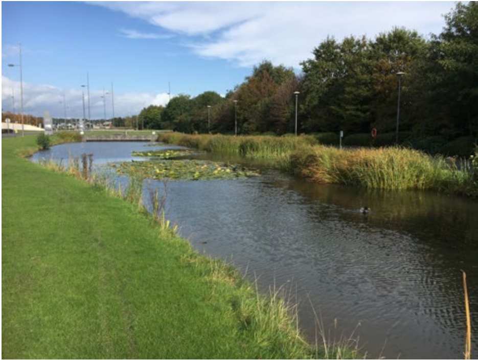
Fig.27 - Example of a Sustainable Urban Drainage System.
