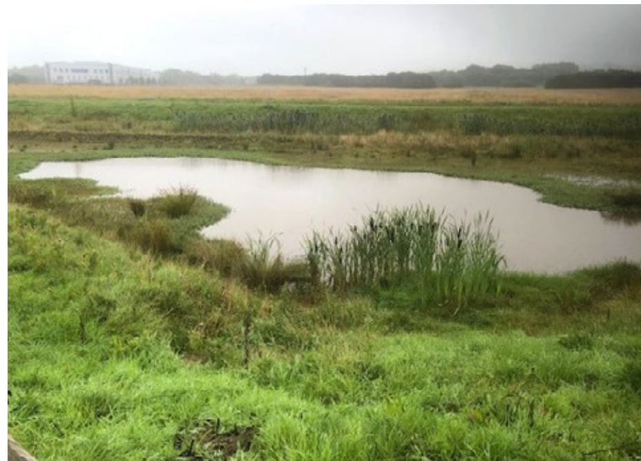
Fig. 32 - SUDS within the SEZ boundary.
