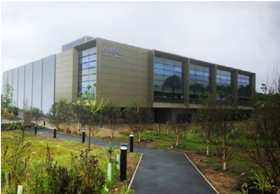
Fig. 30 - Completed landscaping within plots.
