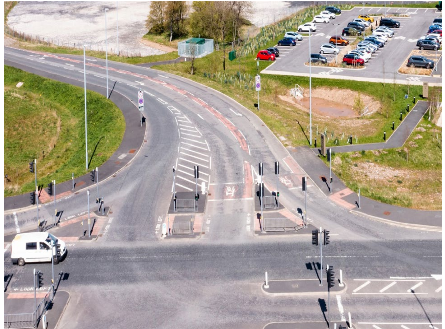
Fig. 34 - Existing photograph of the A677 junction.
