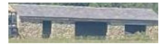
The photos provided show that the repaired building remains the same size. However, instead of using red brick, which previously made up approximately 50% of the structure, natural stone was used during the repair work to ensure that the building visually matched with neighboring properties and that the rural character of the area was not compromised.
