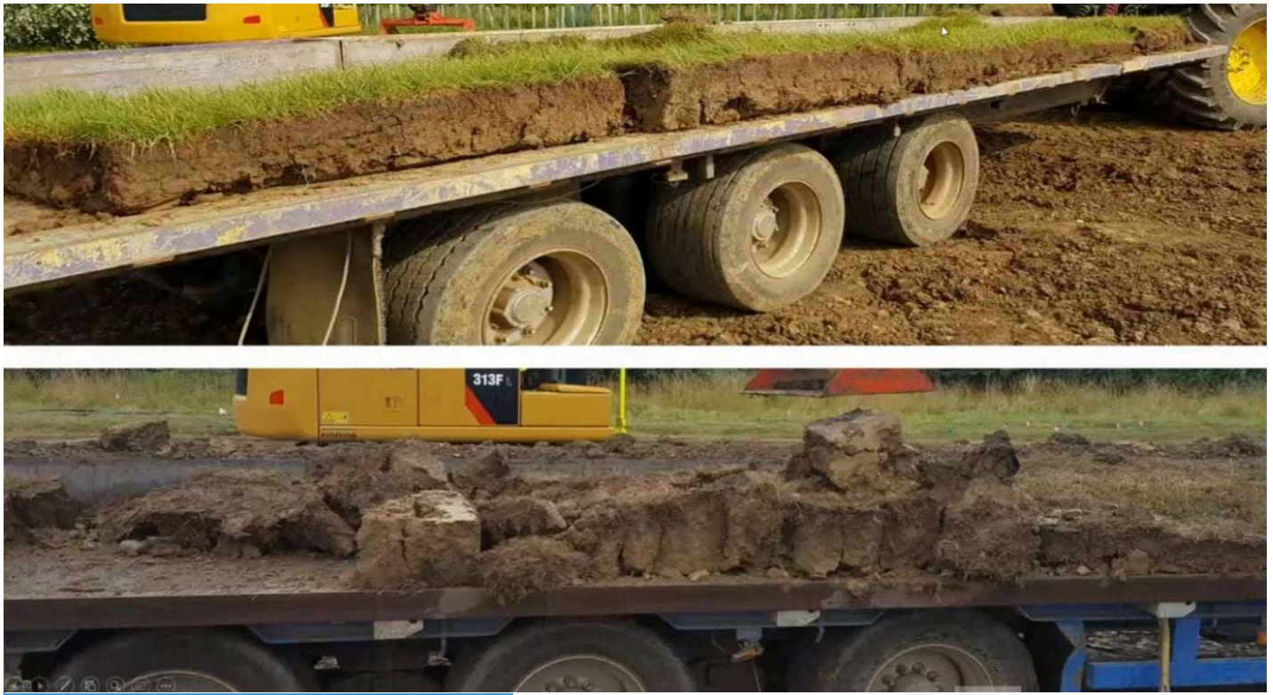
Figure 5 : Difference between turves taken in good weather conditions (top) and those taken in less ideal conditions (bottom) showing the effect on the integrity of the soil and root systems.
