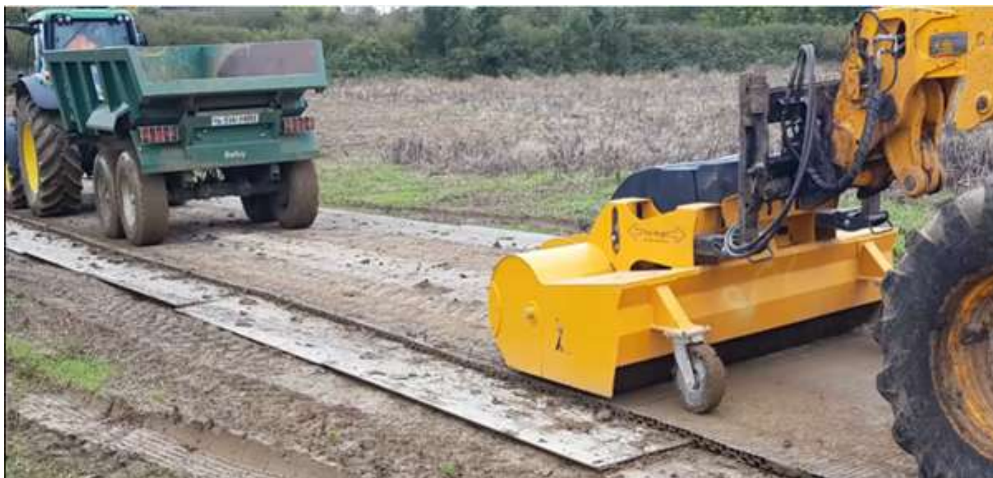
Figure 13: Double track matting used to improve winter access.
