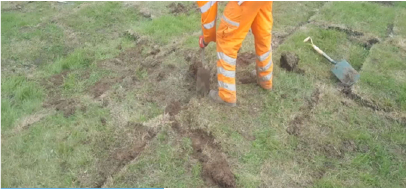
Figure 10: Manual filling of cracks between turves due to earlier drying out, using loose soil from donor. site
