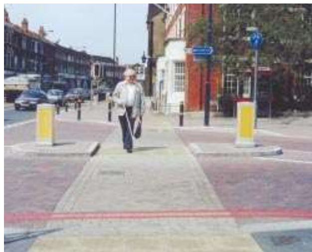
Entry treatments are common on roads joining Red Routes in London. Courtesy: TDFL.
