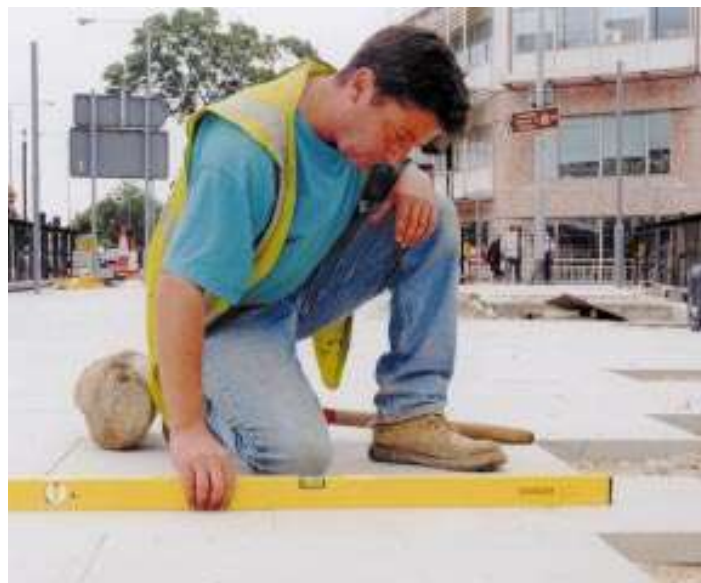
Improving the footway with high quality surfaces – laying York stone paving in London.
