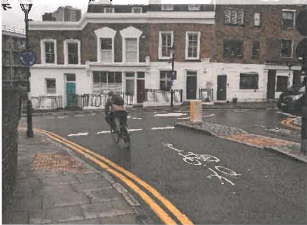
Figure 10.46: Mini-Roundabout on designated mixed traffic cycle route, London
