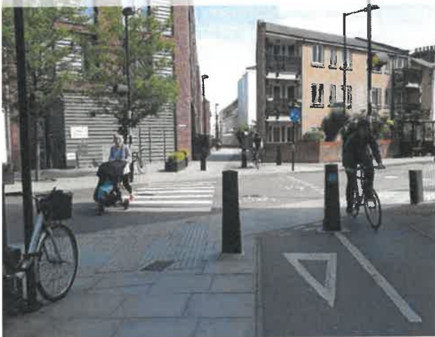
Figure 10.7: Parallel crossing, Hackney
