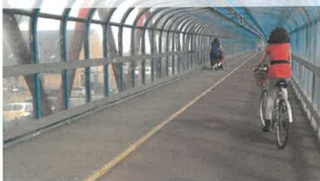
Figure 10.50: Covered pedestrian/cycle bridge across railway tracks, Cambridge
