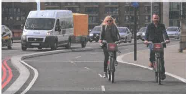
Figure 6.7: Footway level cycle track with raised trapezoidal strip, London
