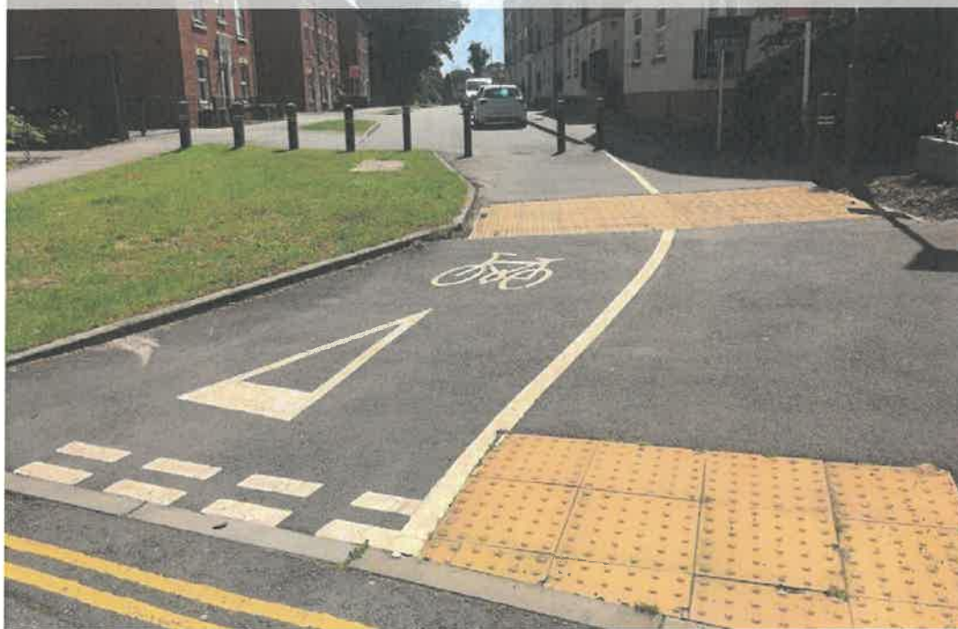
Figure: Example of off-road cycle track along line of a footpath, that crosses the footway to join the road. This type of route can also cross minor roads with priority for the cycle track, using a flat top road hump. (Photograph by Adrian Lord)
