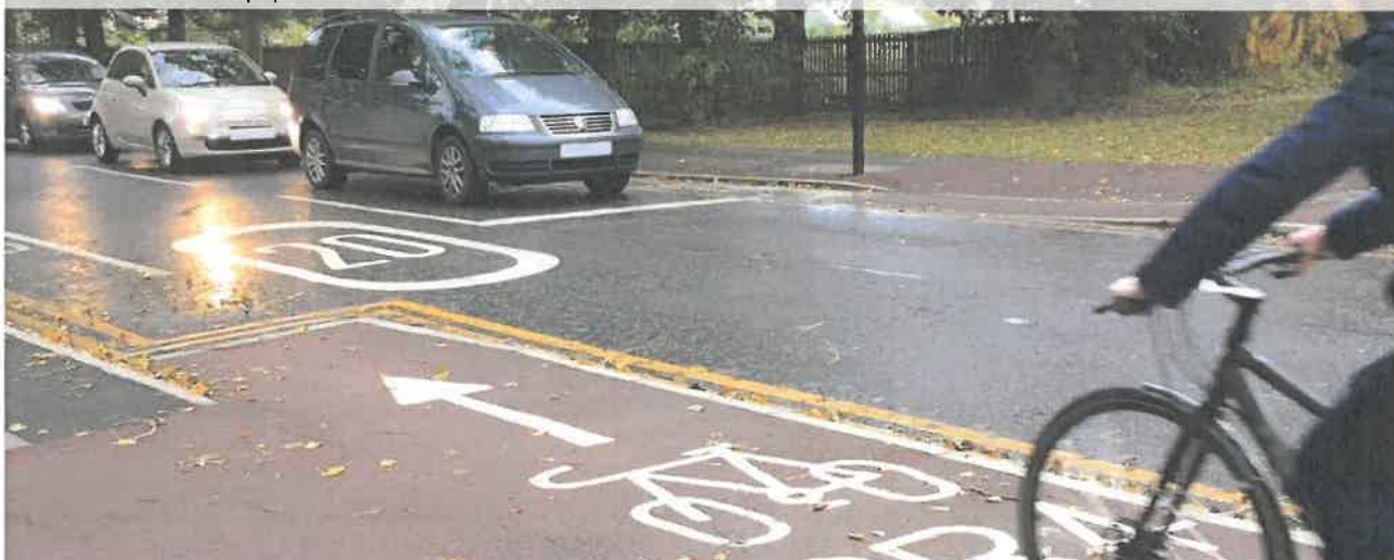
Figure 9.2: Cycle track entry and exit ramps at a signalised junction, Newcastle (Note: double yellow lines not required across transition ramps)
