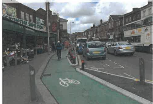
Figure 1.10: Example of kerb-segregated cycle track
