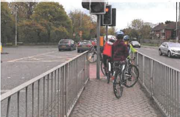
Figure 10.8: Toucan crossing with stagger – can be highly problematic
