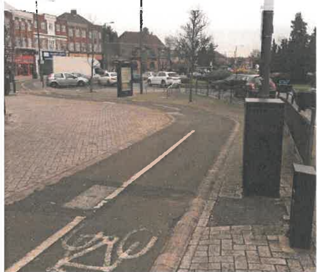
Figure 10.36: Footway-level cycle track around large roundabout, Harrow
