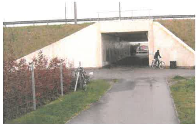
Figure: 10.52 Underbridge (cycle and pedestrian-only) with divided carriageway above to create opening – Lund, Sweden
