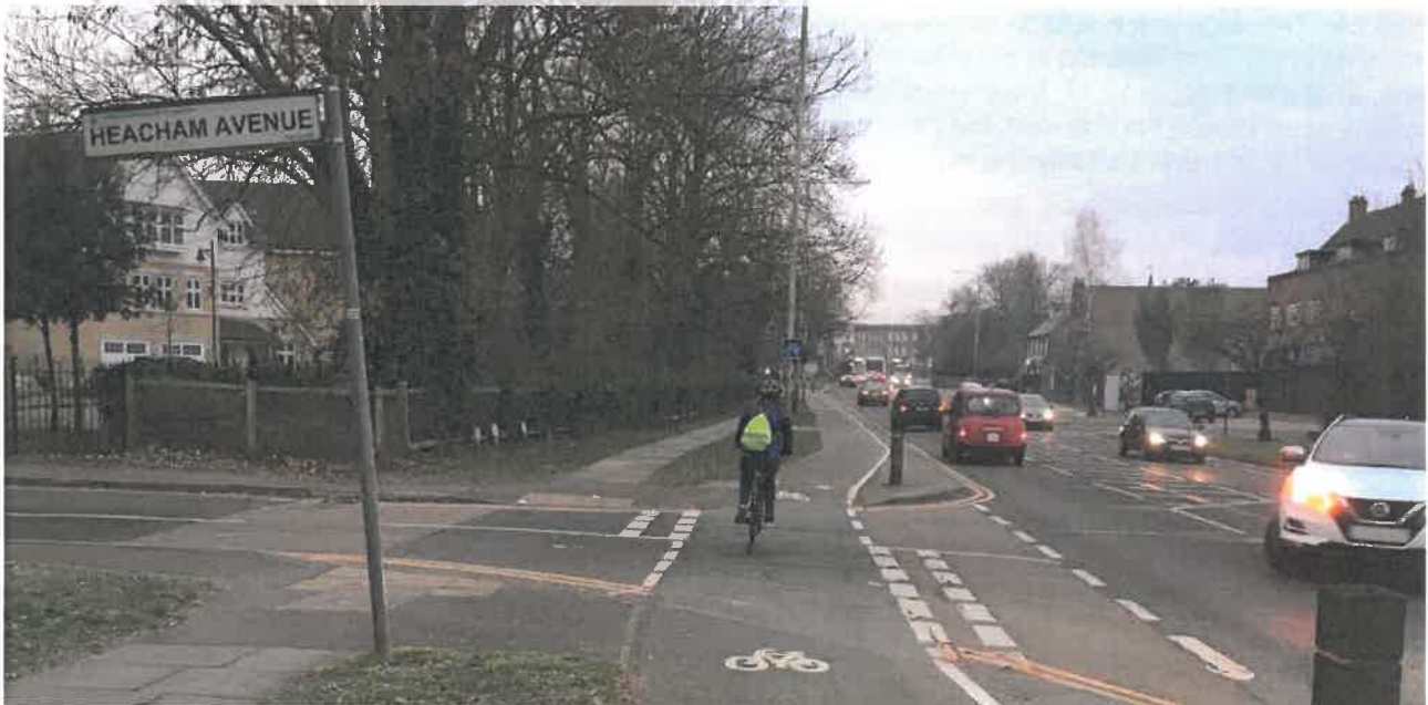
Figure 10.16: Partial set back, marked priority crossing, Hillingdon
