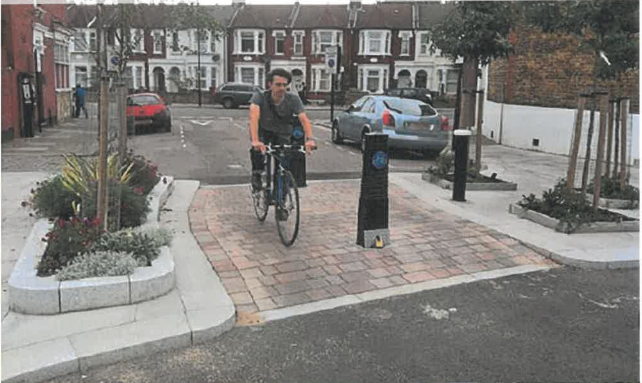
Figure 7.1: Simple modal filters can reduce through traffic while retaining cycle and pedestrian access. The central position enables kerbside car parking to be provided without blocking the facility, and the lockable bollard enables emergency access, Haringey.
