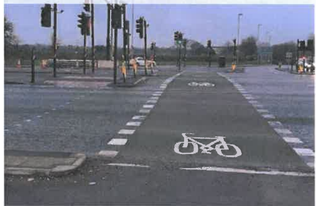
Figure 10.9: Single-stage straight-over cycle crossing next to multi-stage staggered pedestrian crossing, South Gloucestershire
