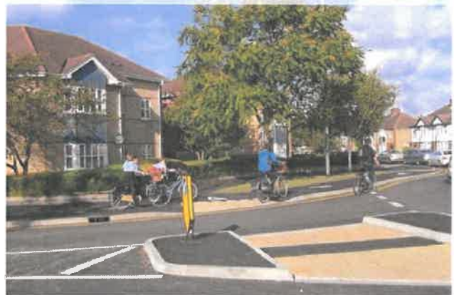
Figure 10.44: The Perne Road Roundabout in Cambridge after remodelling to compact geometry
