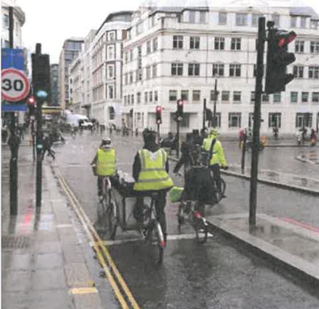
Figure 10.32: Cycle gate, Southwark Bridge, London
