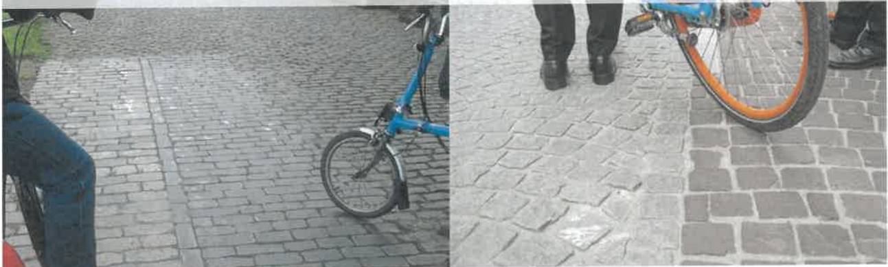
Figure 7.9: Trial site in Bristol to provide smoother surface, and similar application in Bruges with setts in a different colour from the adjacent traffic lane.
