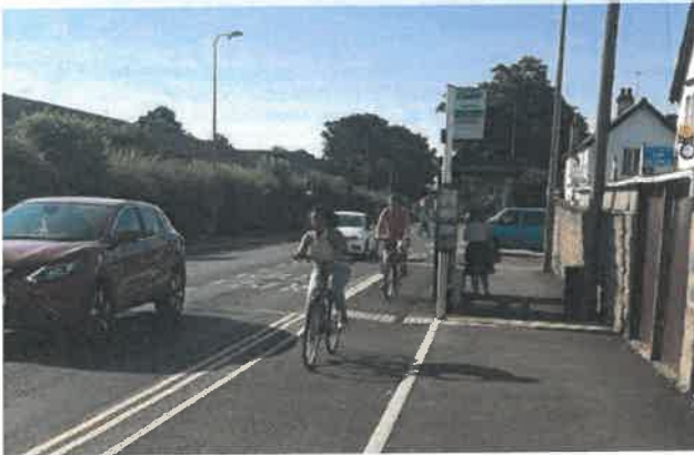
Figure 6.31: Bus stop boarder at quiet suburban bus stop, Oxford
