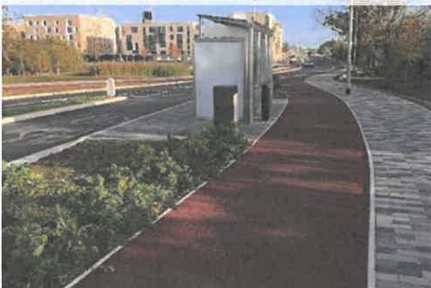
Figure 14.4: One way footway level cycle track past bus stop, North-West Cambridge development.
