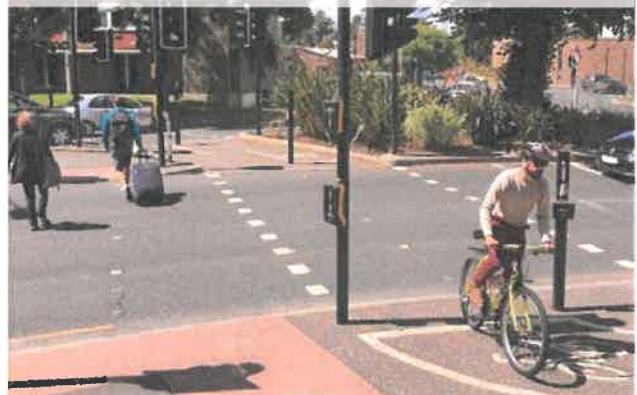
Figure 10.10: Two-stage angled crossing with cycle signals on the central island (Norwich)
