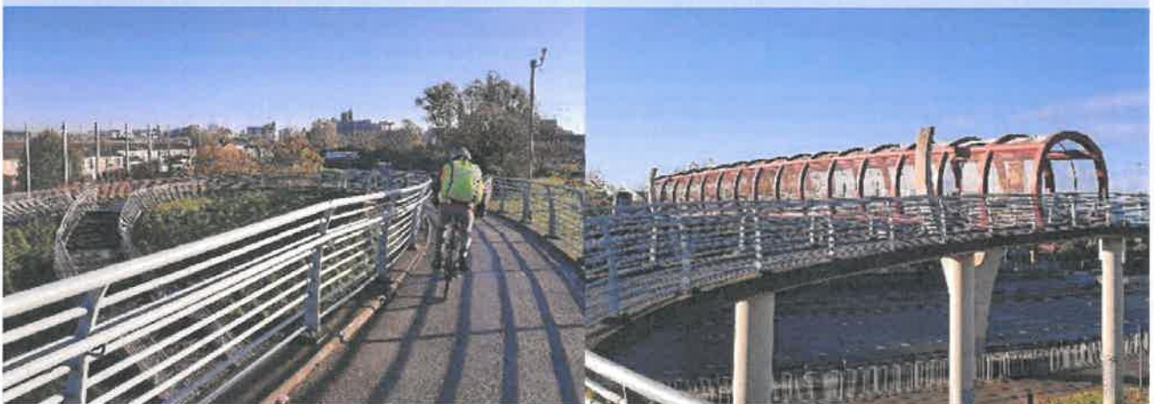
Figure: 10.53: Overbridge with curved ramp approach, Belfast
