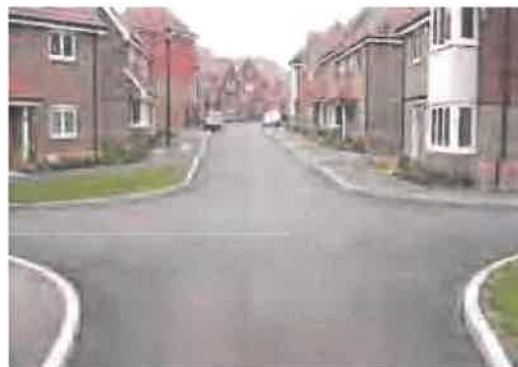
Figure 9.5 Four-way junction with no marked priority.
