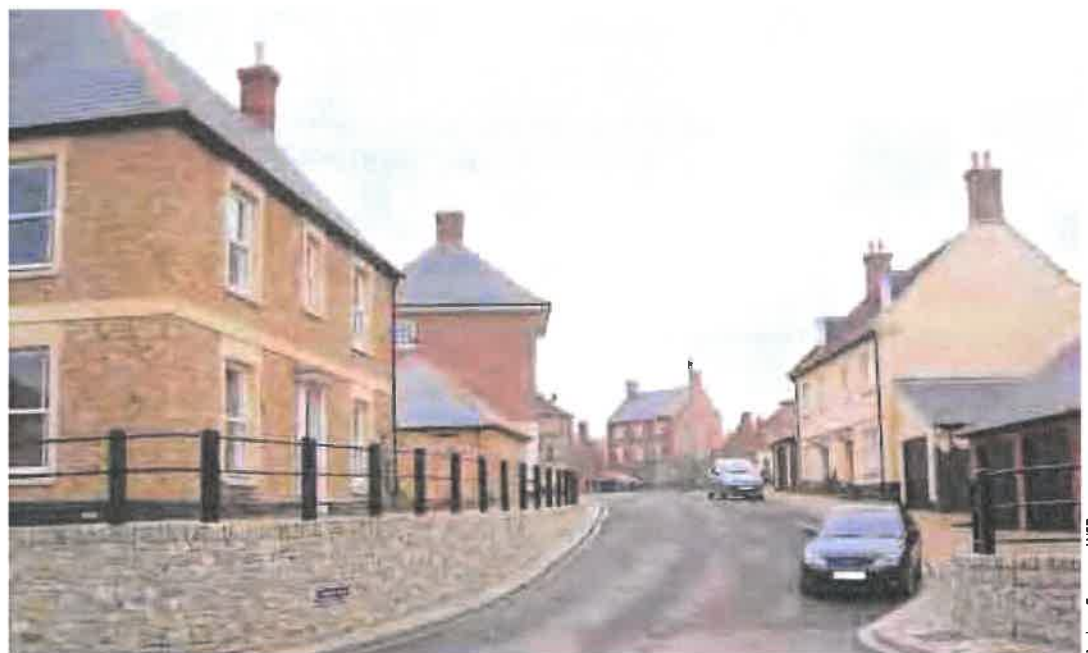
Figure 6.11 In some instances it may be possible to keep footways level when the carriageway is on a gradient, although this example deflects pedestrians wanting to cross the side road significantly from their desire lines.
