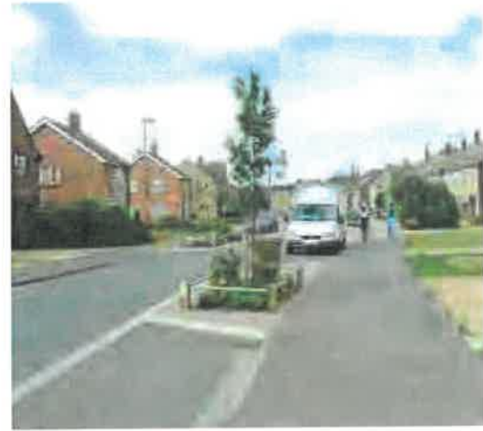
Figure 9.4 Kerb build-out defines parking area and provides room for planting clear of the footway.
