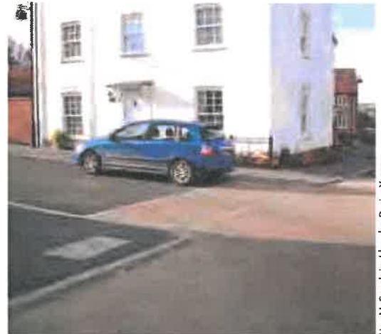
Figure 7.11 Quadrant kerbstones used instead of large radii at junctions reduce the dominance of the carriageway. This is reinforced by the placement and form of the adjacent buildings and the absence of road markings. However, note the lack of dropped kerbs and tactile paving.
