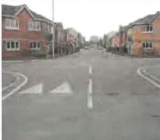
Figure 7.13 Raised tables at junction in Hulme. The table has been raised almost to kerb height.
