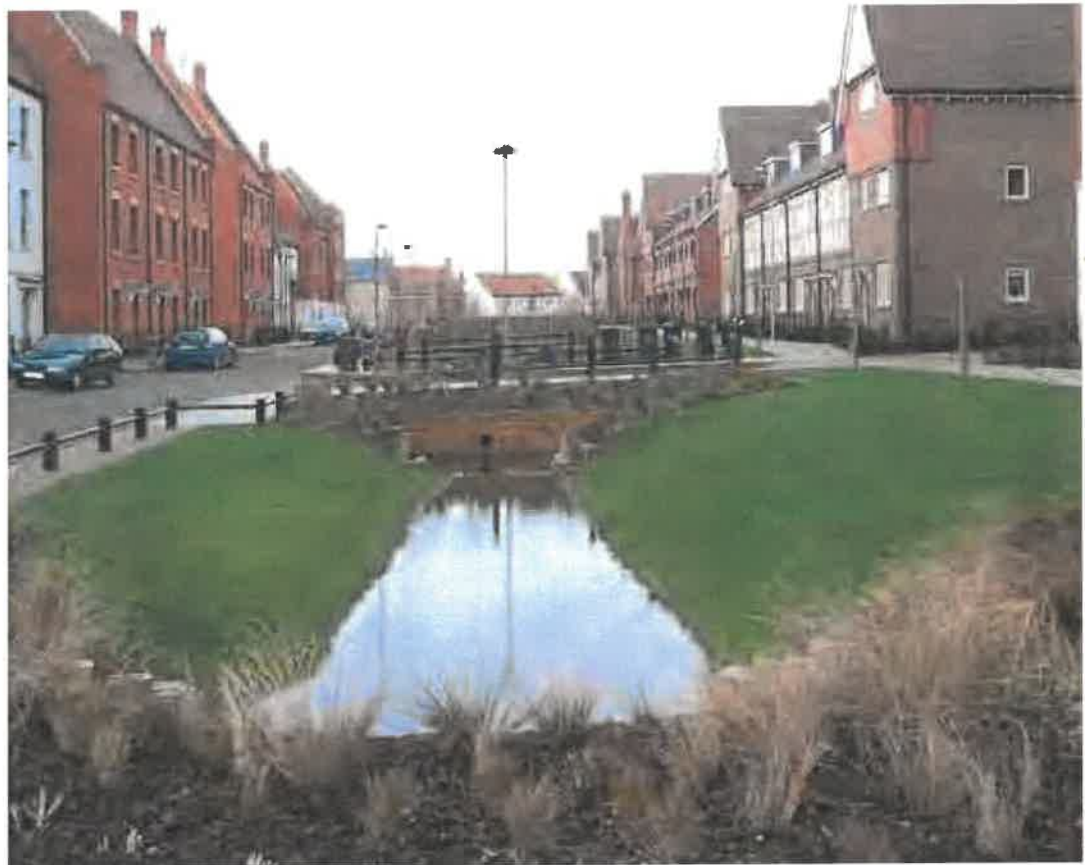
Figure 11.5 Sustainable drainage systems can form an integral and attractive part of the street.
