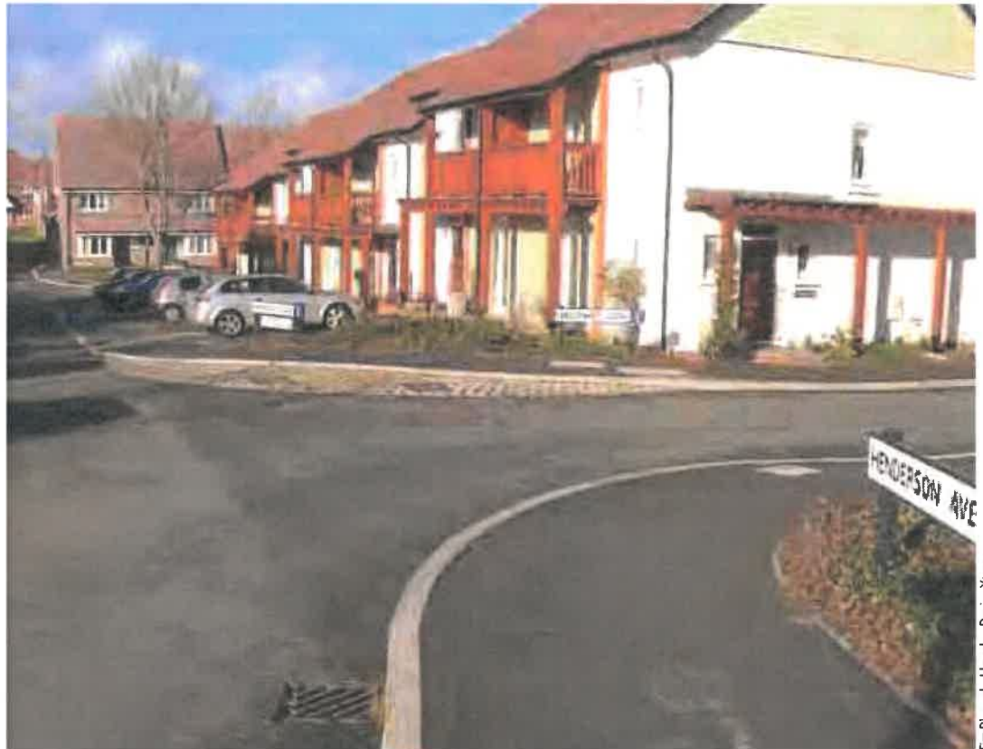
Figure 7.25 The overrun area at this junction is hazardous for pedestrians and/or requires them to divert from their desire line. Notice also the unsightly placing of inspection covers. The layout is particularly hazardous for blind and partially-sighted pedestrians.
