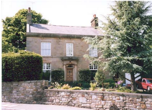
Stone House, Blackburn Road
