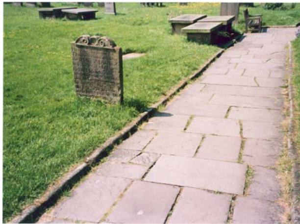
Natural stone paving leading to the south door of St Winifred's Church
