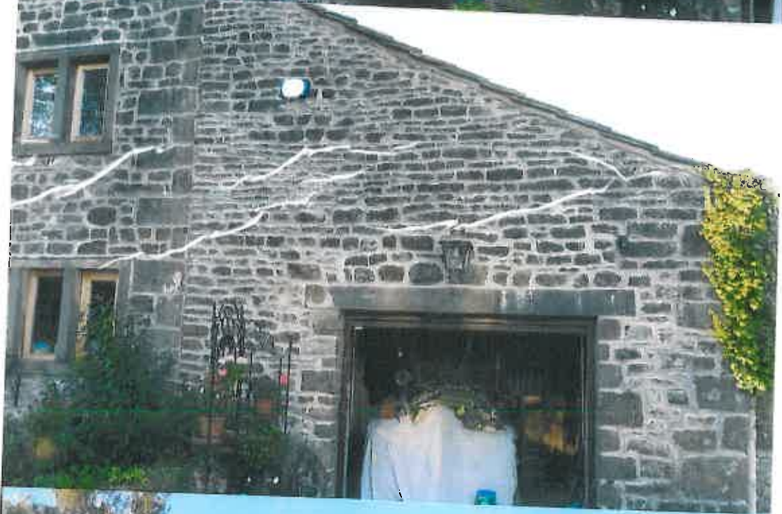
Photo 5 Existing Garage for proposed Conversion
